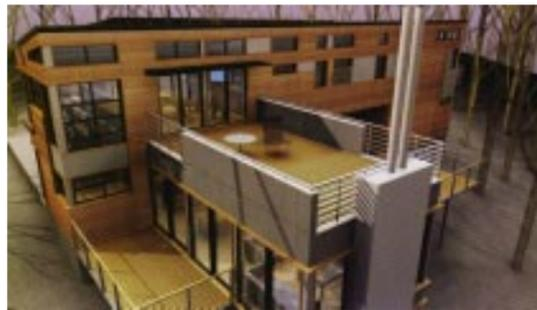
Resolution 4: Architecture of New York City was named the first choice over 12 invited firms by Dwell Magazine for a design for a house to cost \$200,00. The project uses conventional wood framing but uses factory-built modular components in an effort to contain labor costs. It is being built on a North Carolina site.
